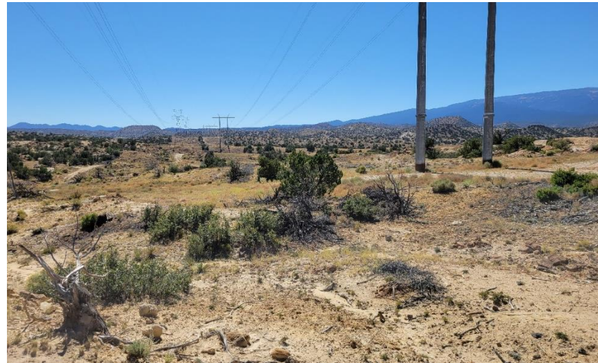
Photo 8 Desert habitat along transmission line corridor, looking southeast.
